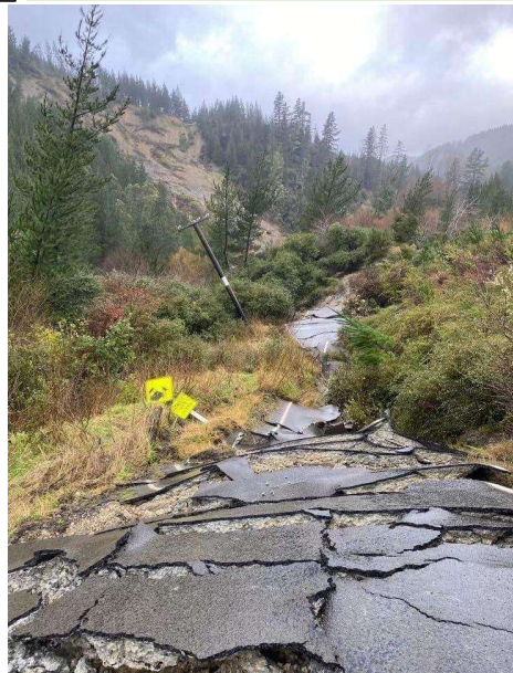
Right: The extent of damage to rural roads and the access issues for the forestry industry, farmers and our rural communities is clear in this image of Tauwharepare Road, Tairāwhiti.
