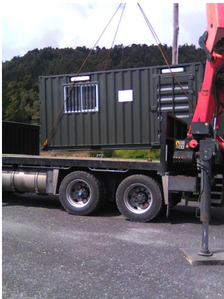
Picture 3 - Container being lifted off truck
