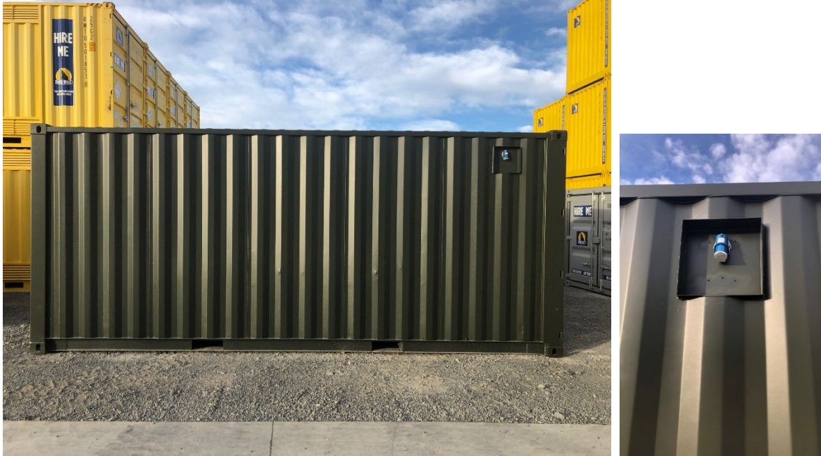
Figure 5 - Rear of container showing power fitting
