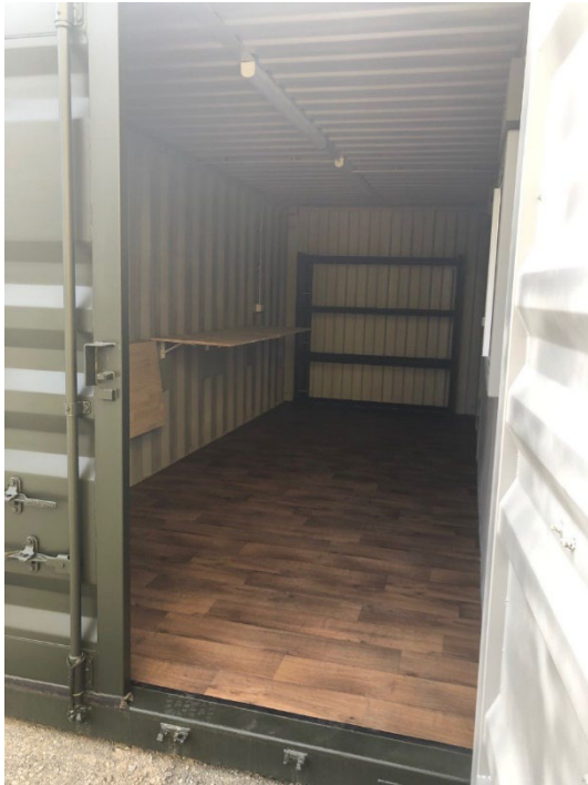
Figure 9 – Side Door open showing inside view of containers showing flooring (and fittings)
