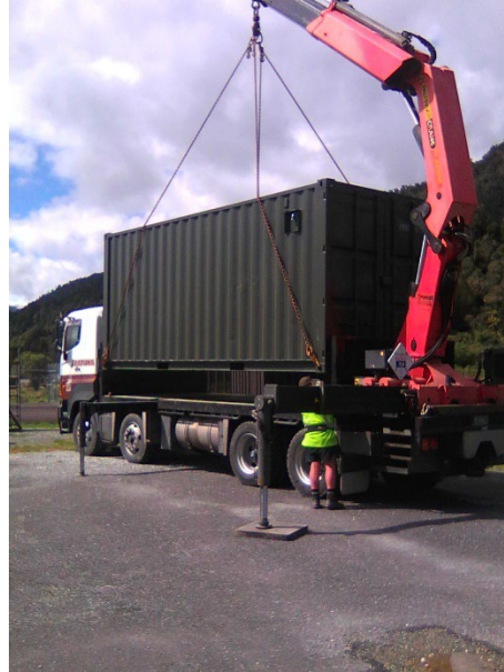
Picture 2 – Preparing container for lift
