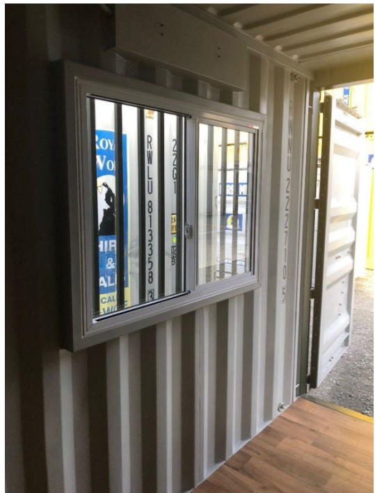
Figure 10 - Window (from inside container)
