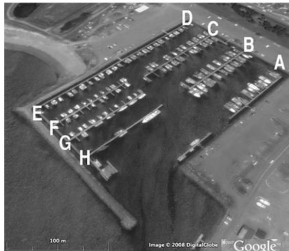
Figure 1.6 Small-boat basin. Docks F, G, and H were either completely or severely damaged during the 2006 tsunami (from Dengler et al., 2008).
