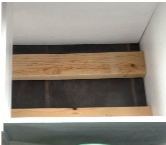
Figure 4.7: Photo of the timber inserts in the base of a compost toilet, these were used to raise the height of the buckets, reduce the gap between seat and bucket and the potential for spills.
