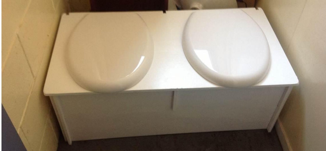
Figure A6.1 Assembled compost toilet unit.
