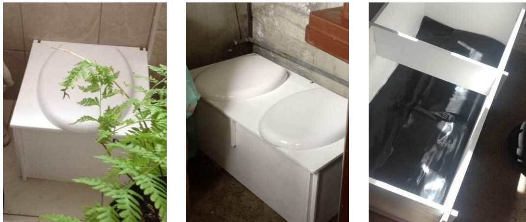
Figure 4.8: The flexibility of the emergency compost toilet. Left: Part of 'split' toilet installed in narrow space in a bathroom. Middle: Compost toilet located in an outside laundry. Right: A lined unit located in spare room of the house.
