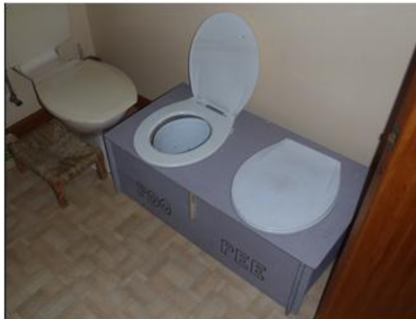
Photo 1: The two-chamber toilet box
