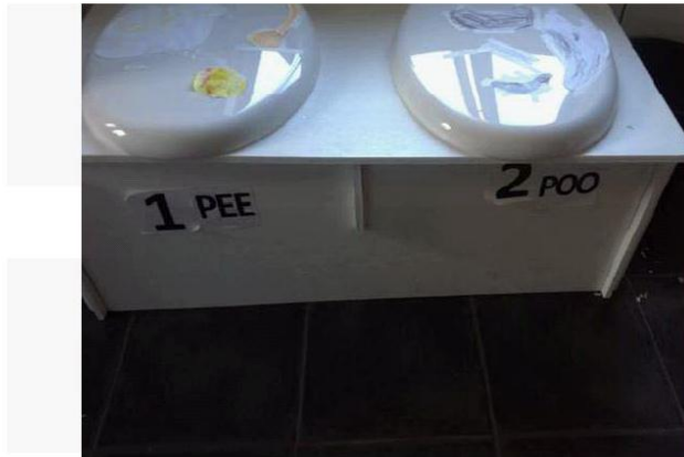
Help to understand what it means to have a compost toilet system.
