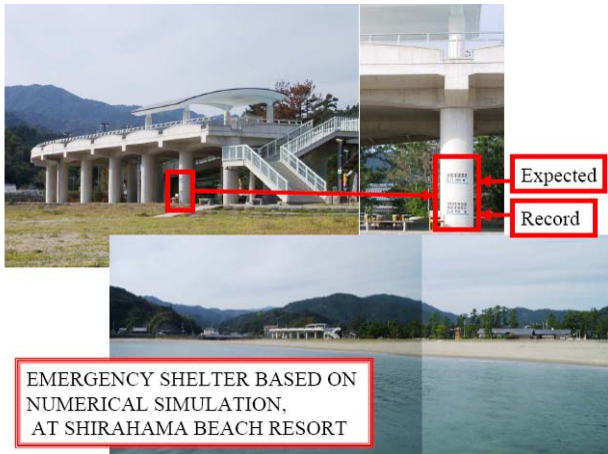
Figure 14 An emergency shelter based on numerical simulation assessment at Shirahama Beach resort, Japan. On the pile of the structure is written the tsunami inundation height expected based on numerical simulation and from the historical record (Source: Shuto and Fujima, 2009).
