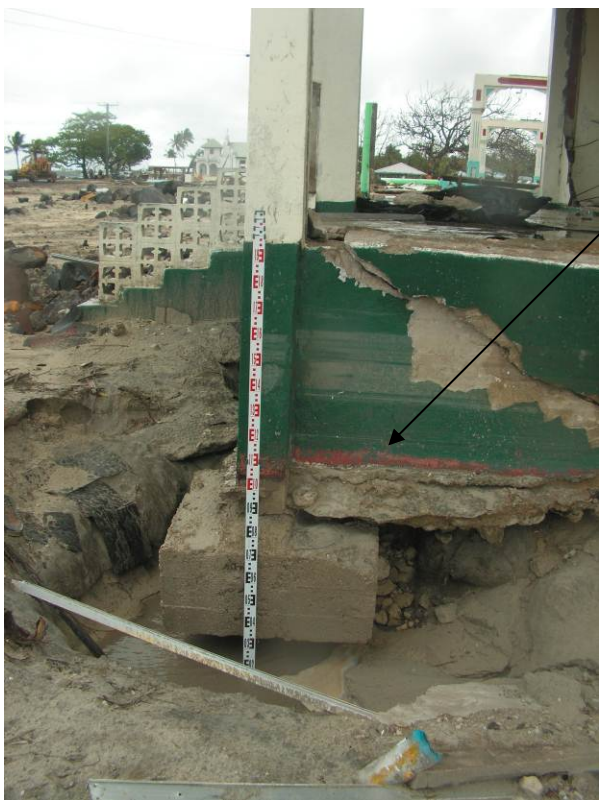
Figure 7 The scouring that typically occurred at the front corner of the building during the December 26, 2004 (Mw = 9.2) at Lampuuk – Lhok Nga Banda Aceh (above) and at Mutiatele - Upolu Island Samoa (below) during the Samoa event (Mw = 8.0). (Photos courtesy: H K Suheimi)
