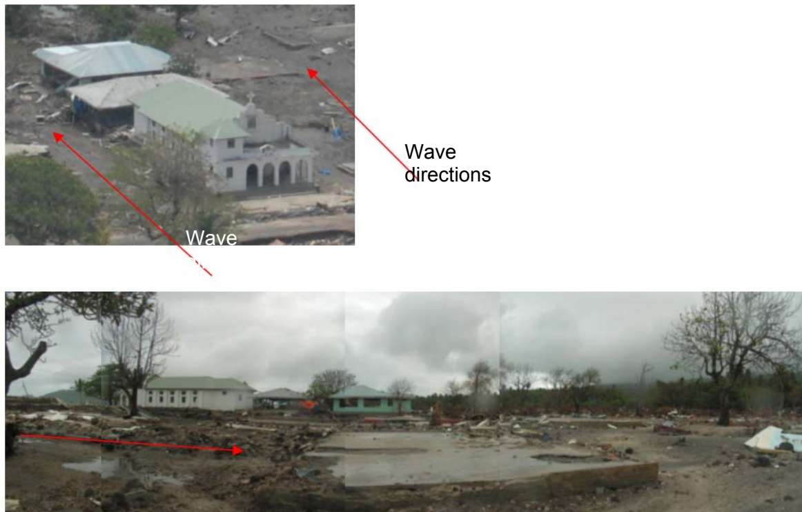
Figure 6 Well-built buildings such as churches, which were located close to the shore, provided a protective function to buildings behind them during the 2009 South Pacific tsunami in Samoa. The flow depth measured at the front of the building is approximately 4.5 m, and the simple houses located behind it were well protected while others were completely wiped out by the tsunami. The red arrows show the direction of the incoming tsunami (Photos courtesy: NZ Air Force).
