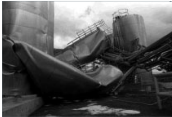
Milk silos at the Edgecumbe dairy factory after the 1987 Edgecumbe earthquake. This earthquake remains New Zealand's costliest to date. Whakatane Beacon .
