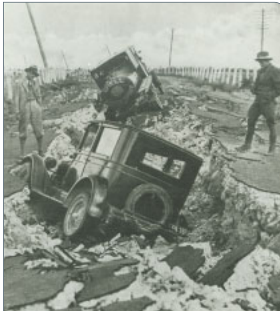
A road after the 1931 Hawke's Bay earthquake. Liquefaction of soil under the road caused it to subside. Hawke's Bay Museum and Art Gallery.
