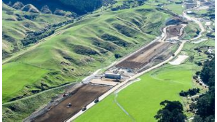
Wellington's Transmission Gully
