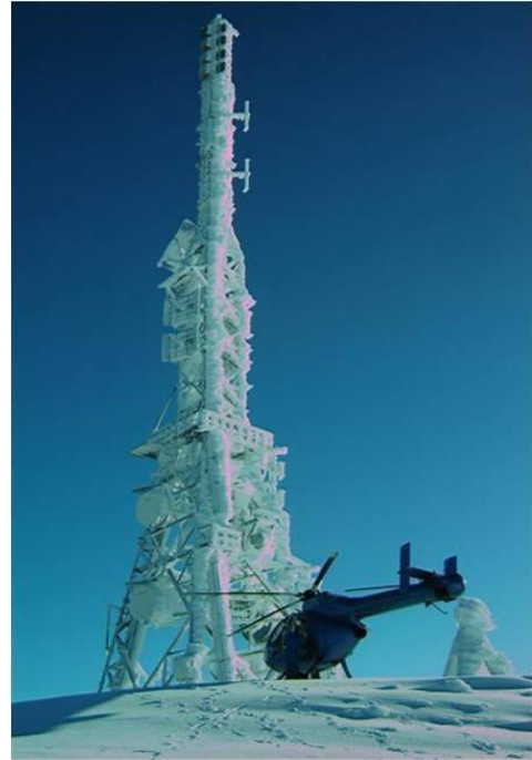
Figure 5-8: A broadcasting tower (continuing to function in ice / snow conditions)
