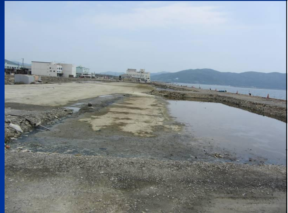
Fill placed to protect land from daily tides in Ishinomaki
