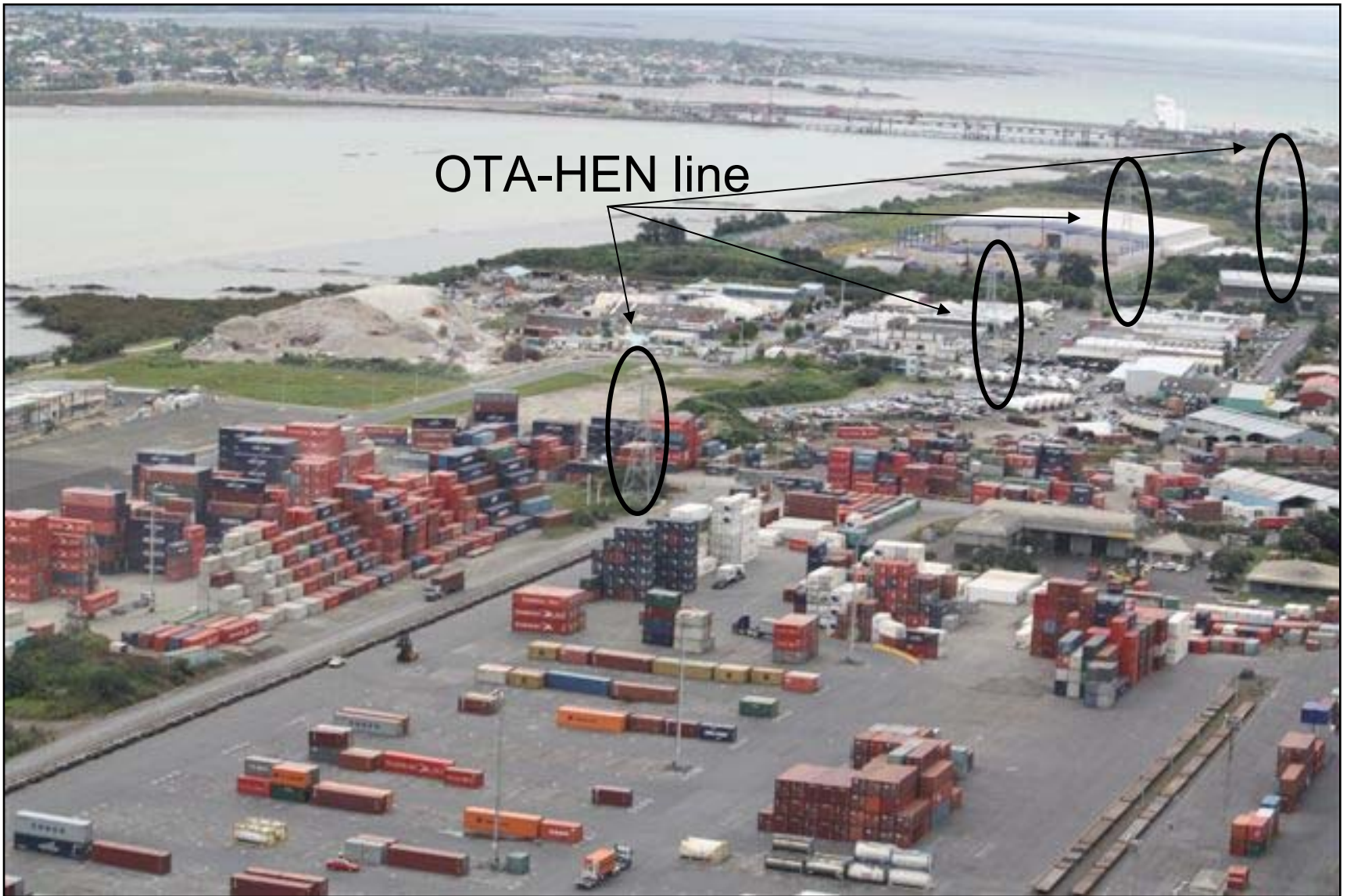
Metrobox container storage yard, Onehunga
