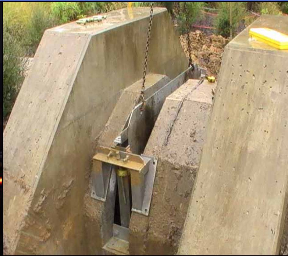
New Stop log during installation
