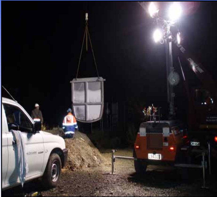
Install stop log to isolate Wairoa Tunnel from upstream system
