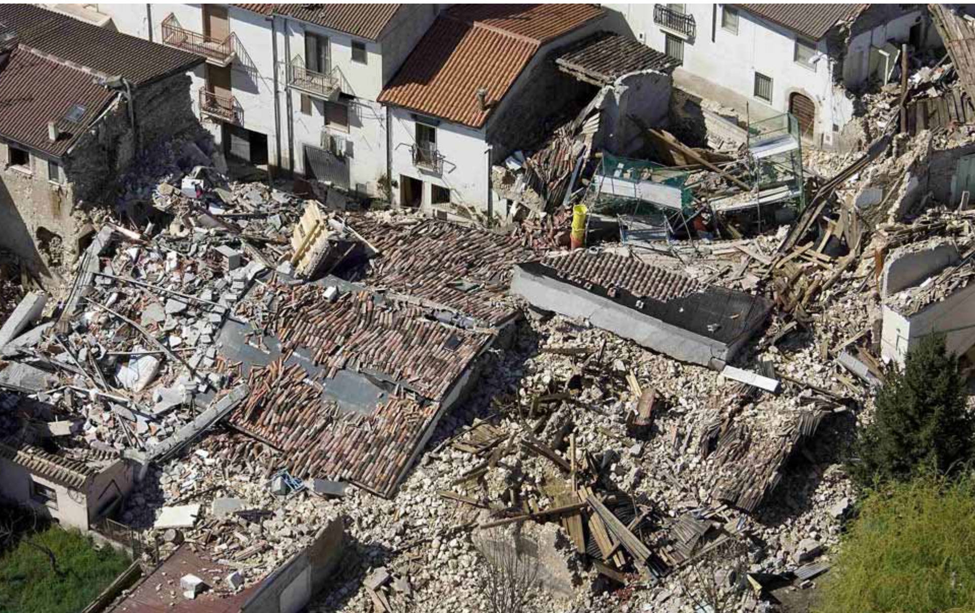
Destroyed houses in the village of Onna are seen in this aerial view near L'Aquila, Italy on April 7, 2009.
