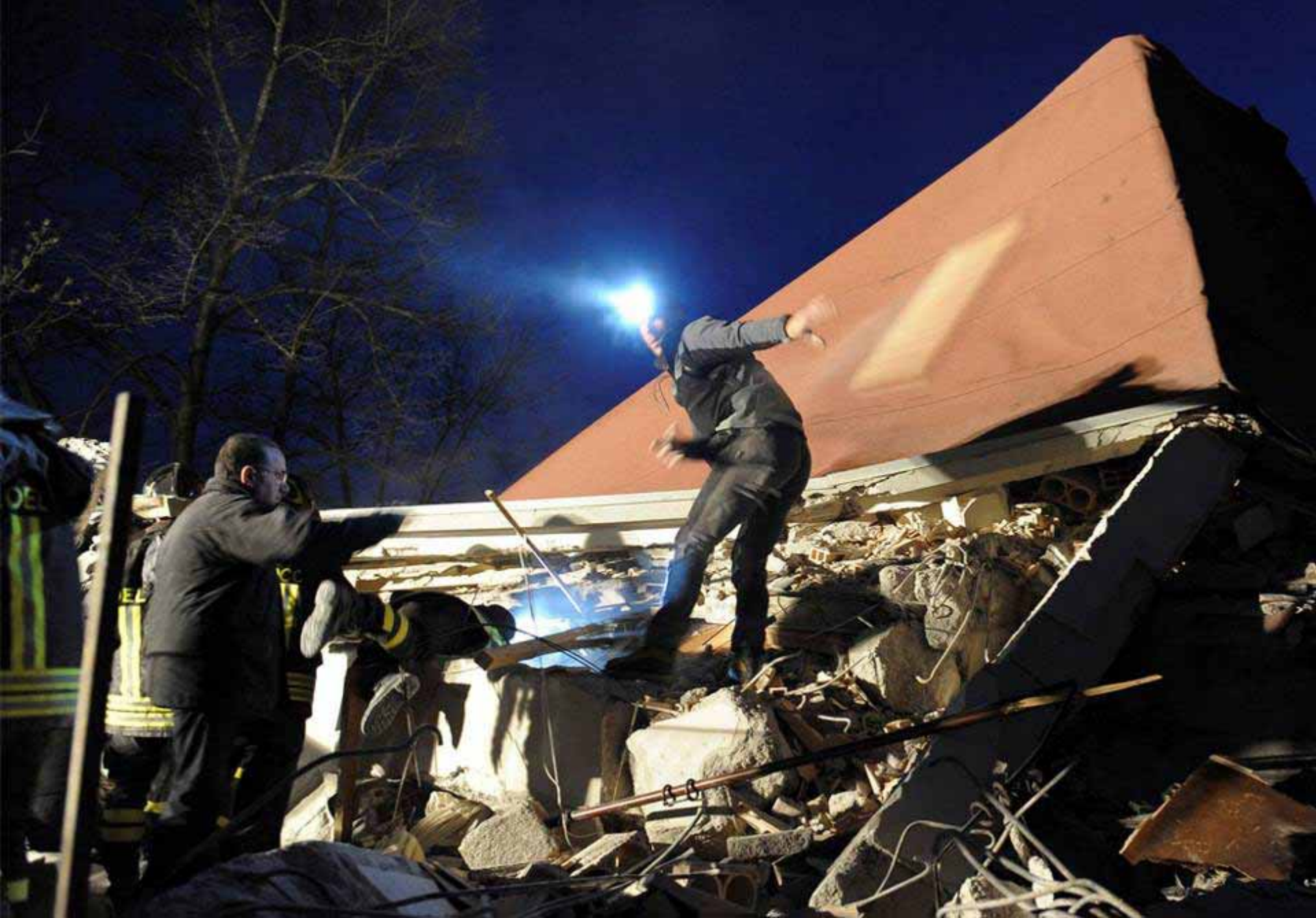
Rescue workers search for survivors under a collapsed house in downtown Aquila April 6, 2009.
