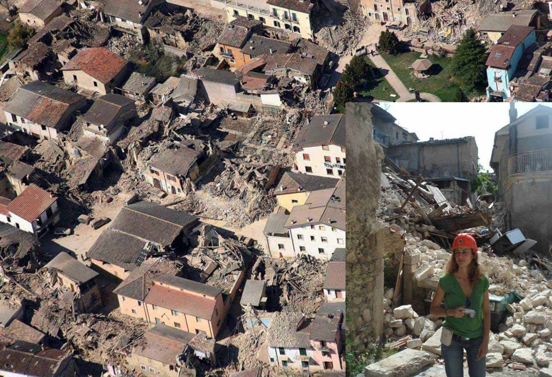
debris from damaged residential and monumental buildings adjacent to the roads
