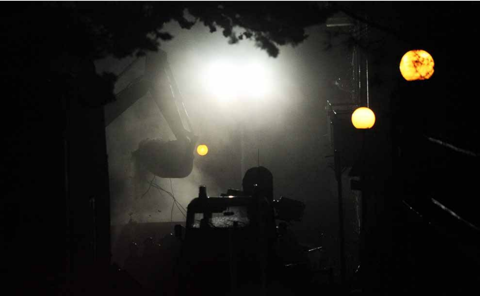
An excavator digs near a collapsed building in Aquila April 6, 2009.
