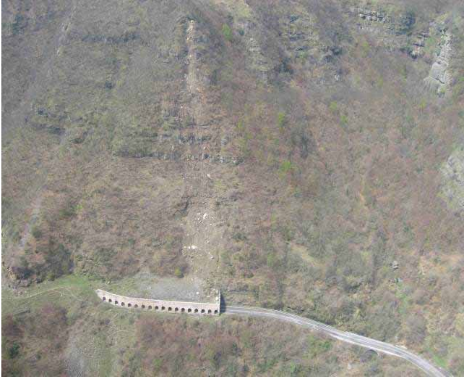
S.S. 80 “del Gran Sasso d’Italia” rockfalls on rock-proof tunnel
