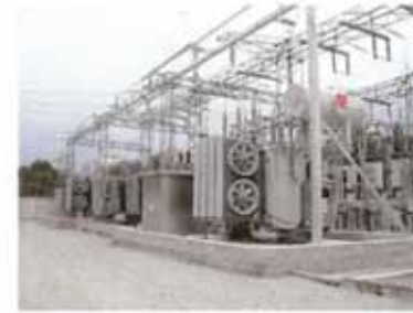
Older lattice and newer pipe gantries
