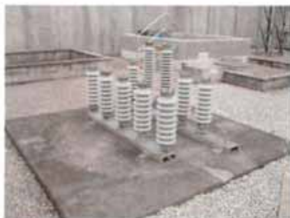
Spares restrained on spares pad
