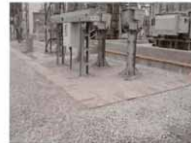
Note CB's and CT's etc on well grouted base plates
