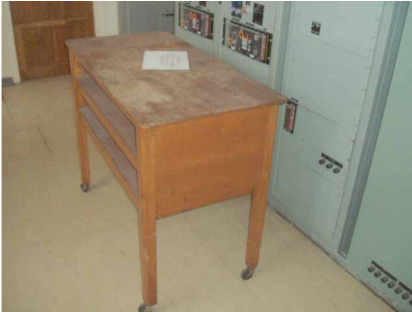
Unsecured wheeled furniture in relay room
