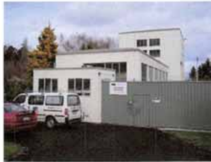
Traditional cast insitu reinforced concrete control building and crane room
