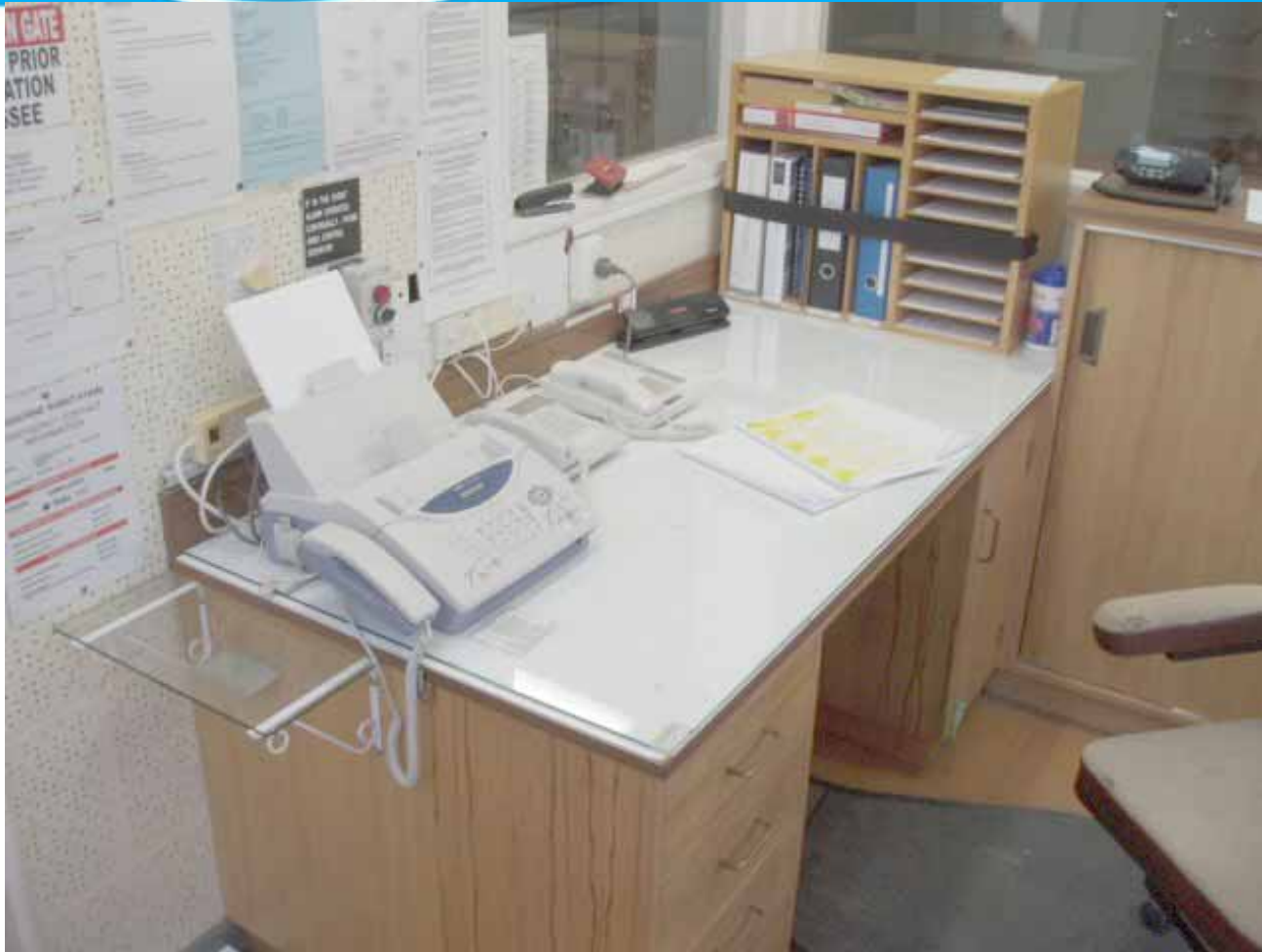
Furniture and equipment restrained (Gisborne prior to earthquake)
