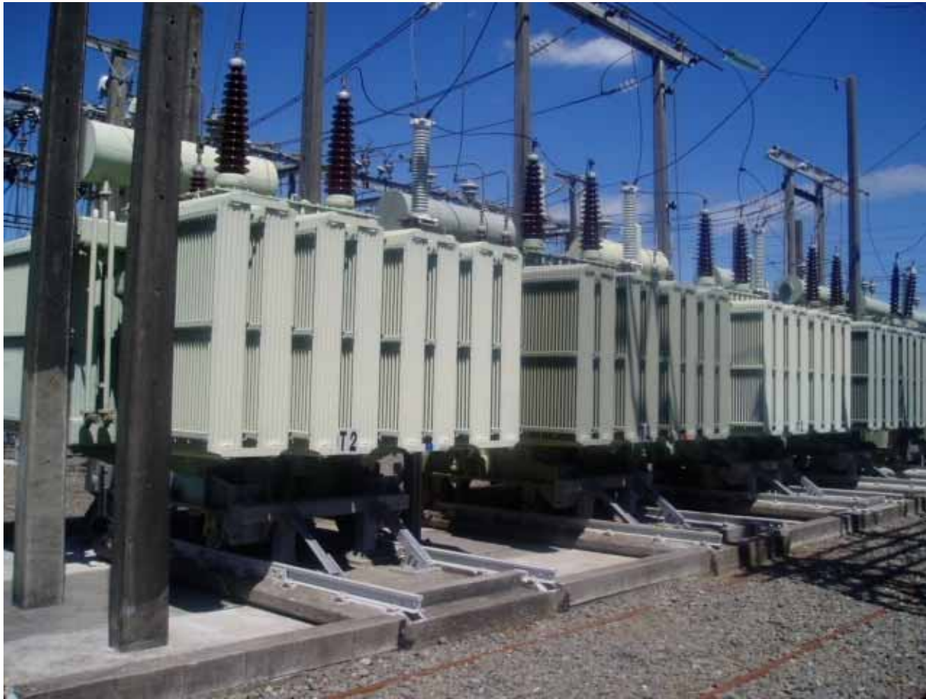
Transformer bank well restrained
