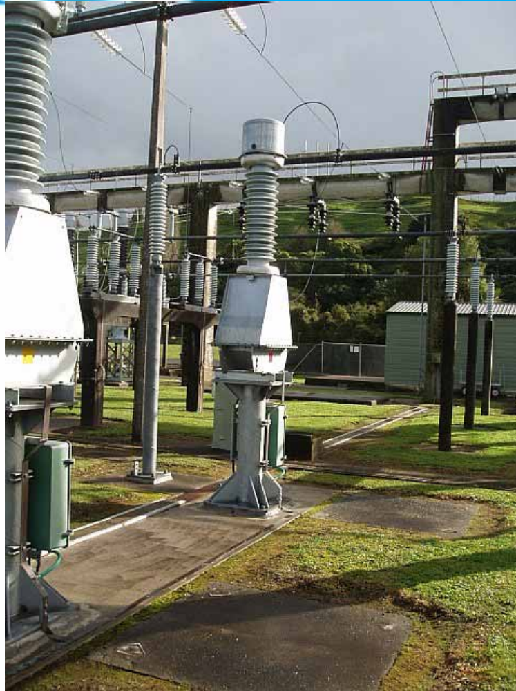
Equipment on robust support stands
