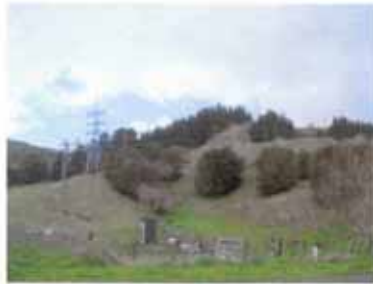
Transmission line feeding Gisborne
