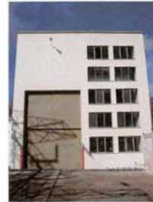
Crane room looking north west
