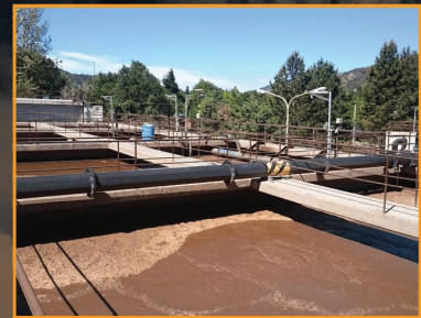
Biological reactors at the municipal wastewater treatment plant at San Martin de los Andes, Argentina, continued to function without problems despite receiving 2 cm of ashfall from the 2015 eruption of Calbuco volcano, 165 km away in Chile. This was partially because the town's storm drains and sewers are well separated, so very little ash entered the plant in raw wastewater. Photo credit: Daniel Blake
